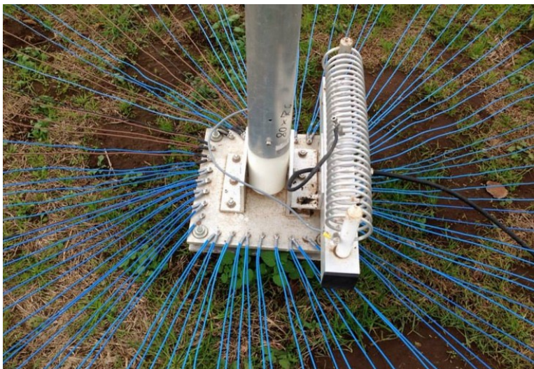
Fig 15: Example of ground plane reinforcement
